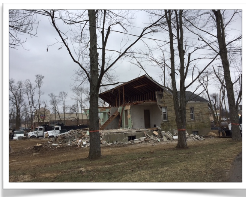
House demolition on Wolf Creek.
